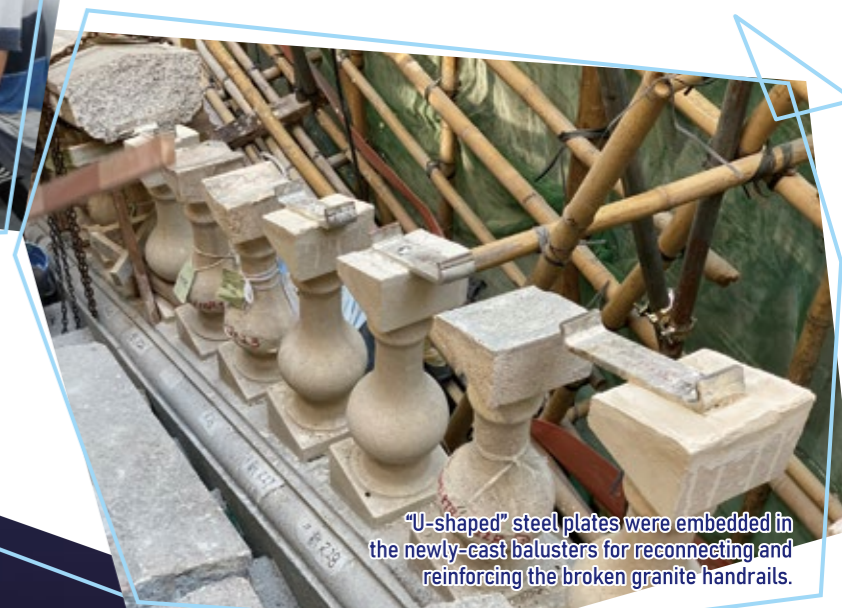
The project's Building Surveyor (middle on the left) inspecting the newly cast balusters.
